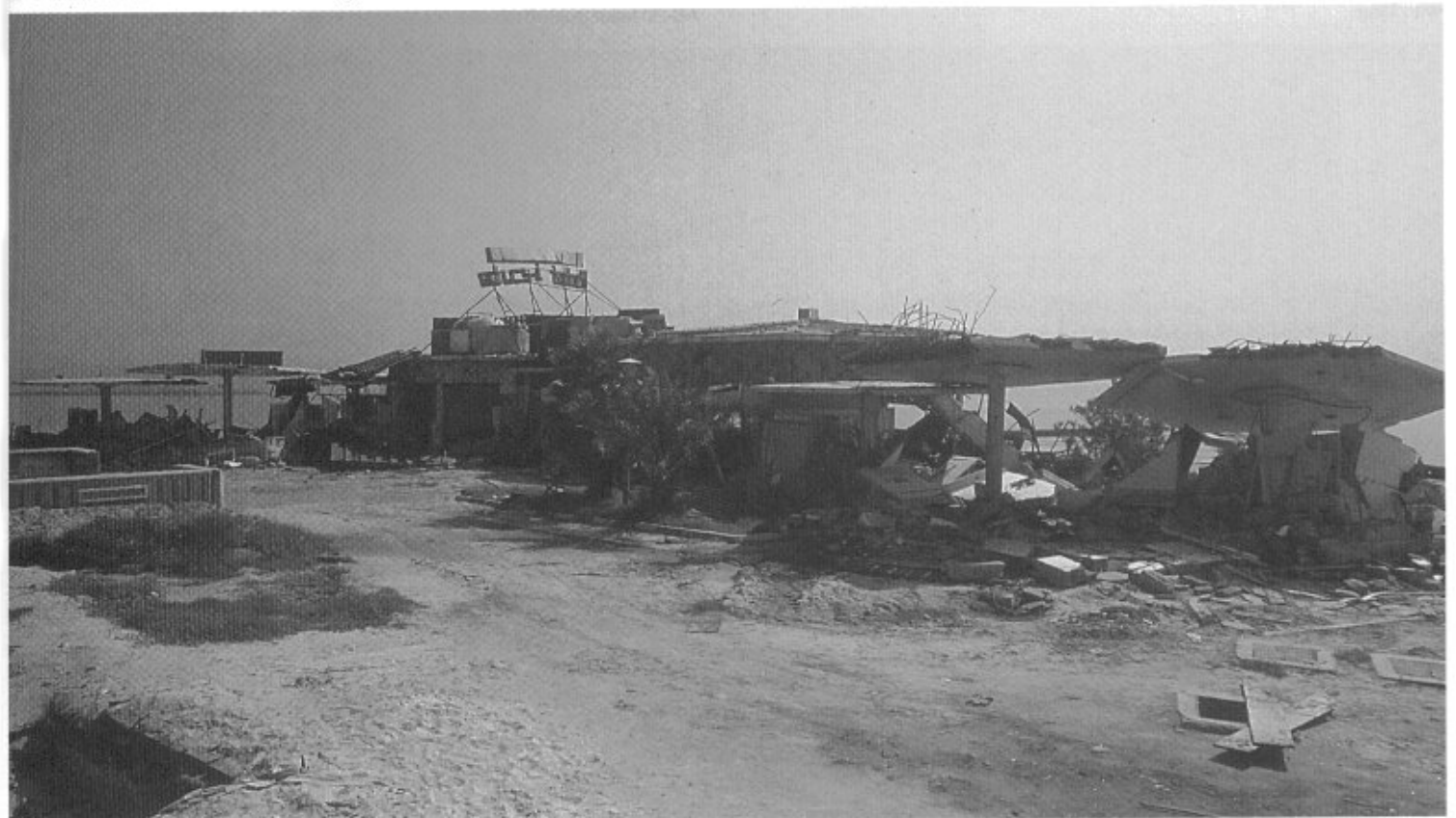
Many restaurants and buildings in Kuwait City were turned into some sort of bunkers and fortifications by the Iraqis. Many were blown up by the Iraqis when they evacuated Kuwait City.
