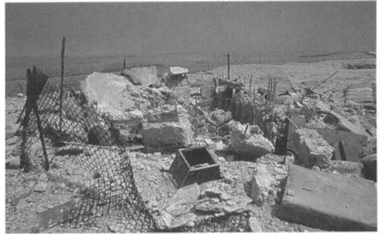
A destroyed bunker in Kuwait City.
