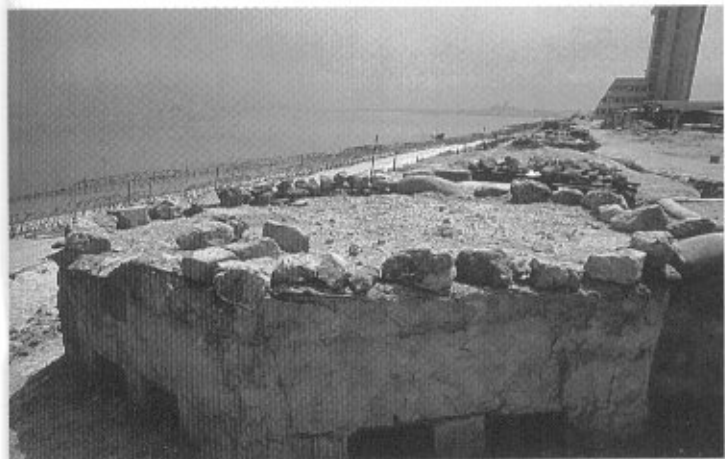
Some bunkers have machine gun apertures, designed to fortify the beachhead in case of a frontal assault from the sea.
